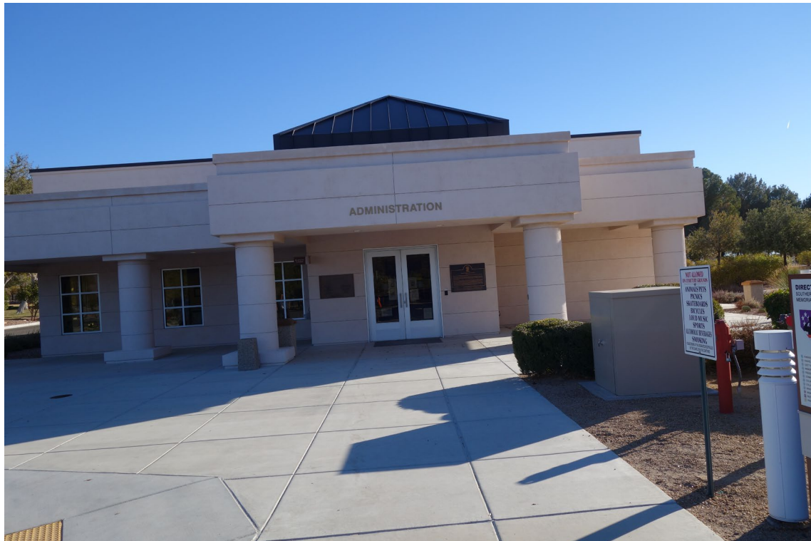
Administration Building – FCA Building #3147 Description: Exterior of the Building.
