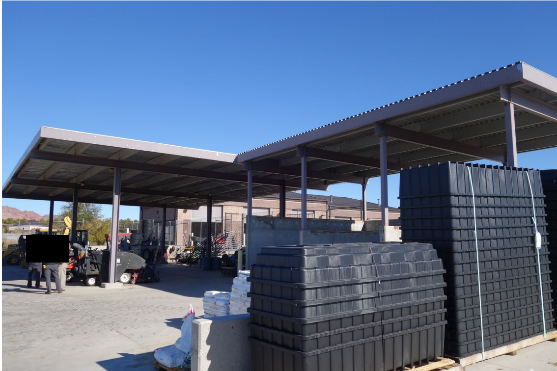
Open Metal Canopy – FCA Building #2998 Description: Exterior of the Structure.
